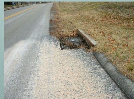
Salt near storm drain
